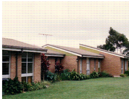
B Block classrooms looking east towards Link Road. Note eucalyptus trees in the background, one of which recently came down on Faith Kindergarten during storms.
