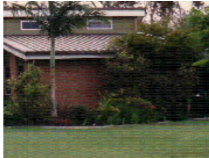
View towards the original Admin Block from Link Road car park entry.
