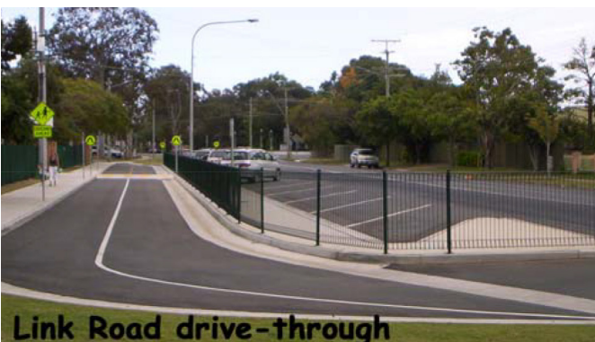
Stage 8 I block Link Road
